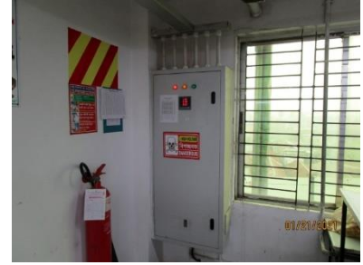
21. Electrical SDB board
